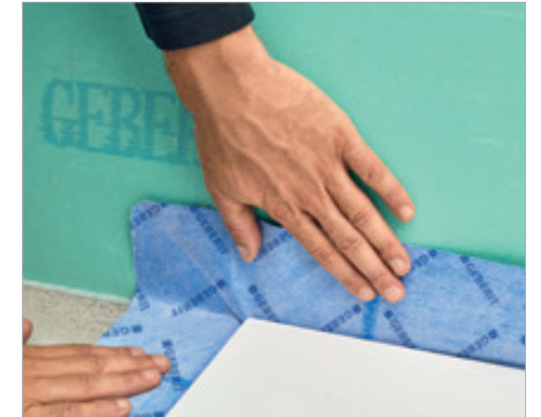
↑ The factory-set sealing fleece saves time and provides a secure seal.
