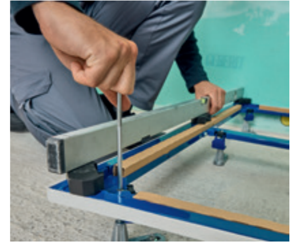
↑ The height of the feet can easily be adjusted from above with an hexagon key, ensuring a floor-level installation of the shower surface.
