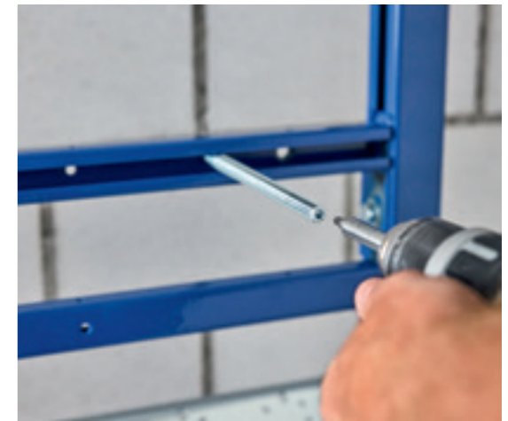
↑ The threaded rods have deep-drawn threads, so they can be screwed in to the required length without needing to cut them to length. You can also use movable T-slot nuts.
