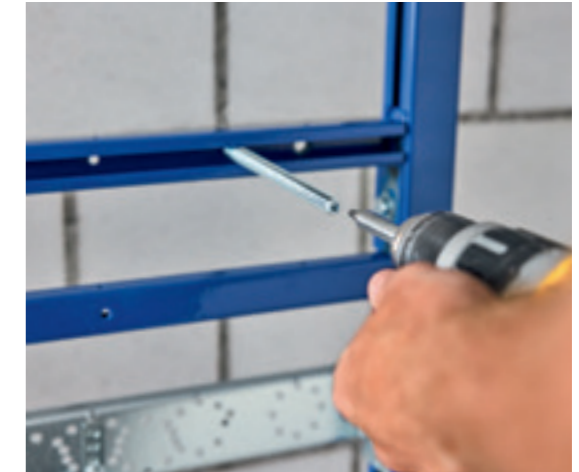
↑ Threaded rods that can be screwed through, even in the washbasin element, remove the need to cut them to length later.
