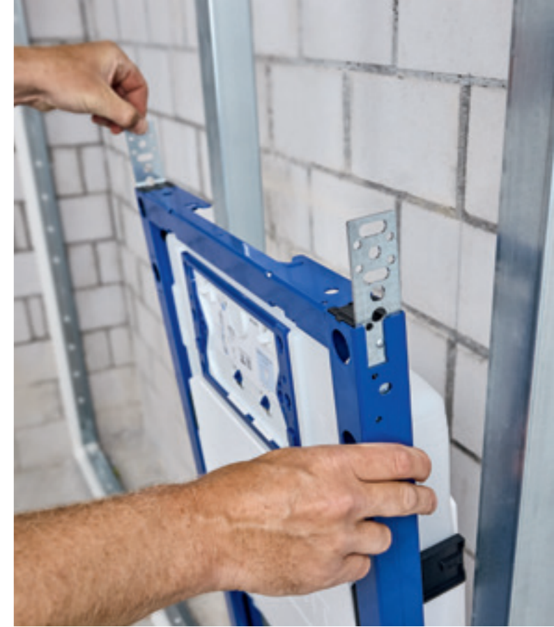
↑ Practical extension for side stud fastening
