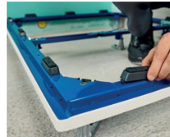
↑ Position the supplied spacers for the steel shower surfaces.
